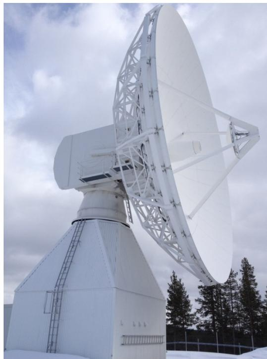
**Figure 3-9: Kiruna 15-m ground antenna (KIR-1) equipped with a *tilt over Elevation over Azimuth* mount to cope with very high elevation passes**
