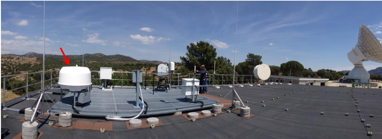
**Figure 3-38: Installed RFI scanning array in the deep space site of Cebrenos (Spain)**
