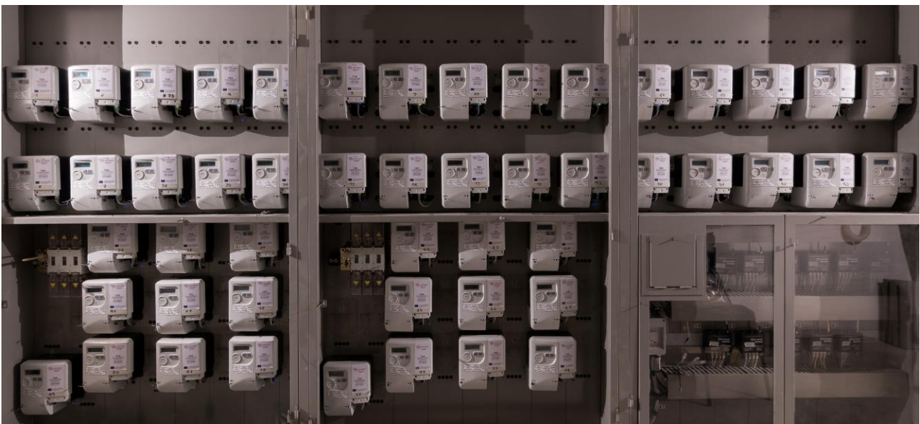
Figure 95. SLAM installation in an apartment building
