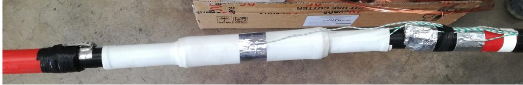
Figure 58. Thermocouple placed above joint materials during the packaging.
