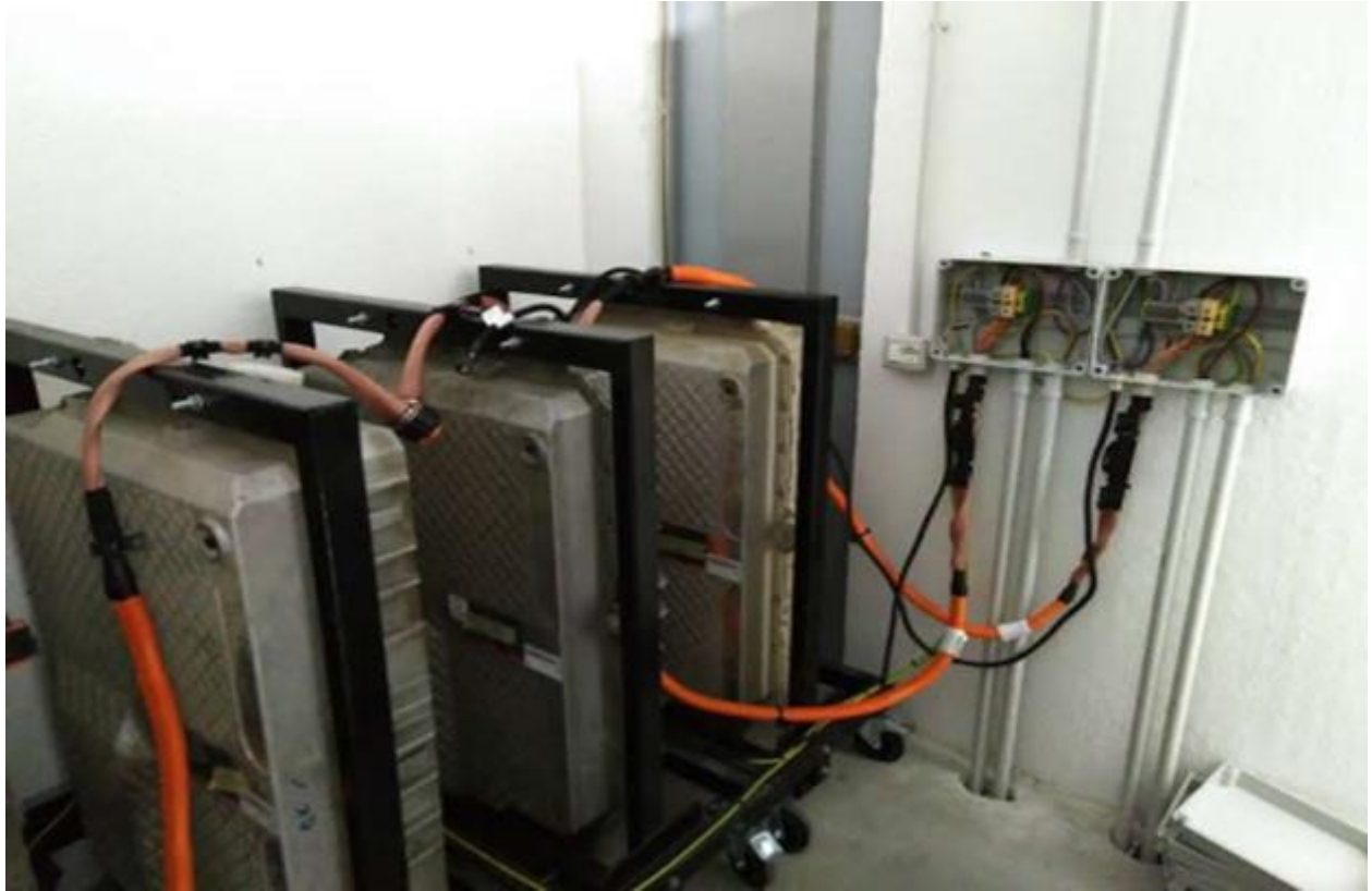
Figure 110. 2nd life Li-ion batteries
