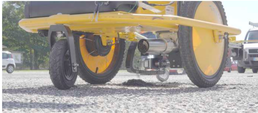
Figure 18. Pothole filling in a pothole.
