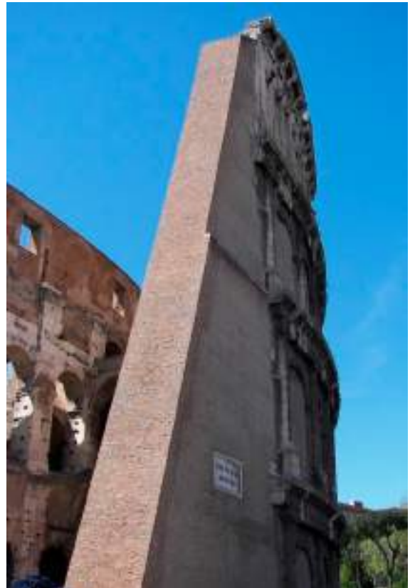
Fig. 41. Colosseo Buttress, Rome. Photo by Susana Mora, 2015.
