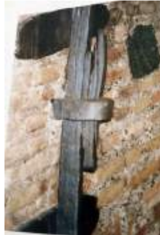
Fig. 62. On the left: Traditional bracing reinforcement. From G. Carbonara, Atlante del restauro architettonico , vol. II, Utet, Torino 2004, p. 565.
