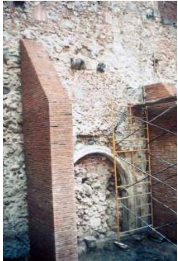
Fig. 39. Buttress, S.P. de Arlanza, Burgos, 1989. Restoration by S.P. Arroyo and Susana Mora.
