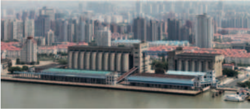
Fig. 9. Grain silos in Minsheng Road in Shanghai / I silos di grano lungo Minsheng Road a Shanghai
