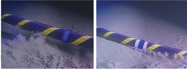
Fig. 1. Submarine cable laying above the water–seabed interface (Courtesy of Nexans).
