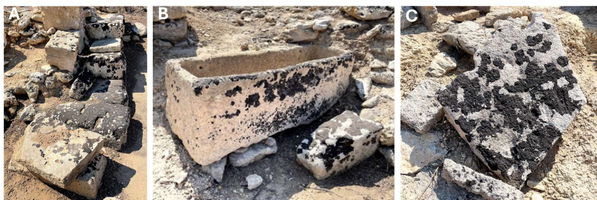
Figure B2.1. Calcarenite walls covered by black lichens (A-C) Motya Island
