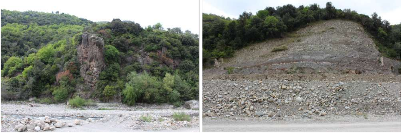
Figure 50: a) cliff made of breccias of the second lithofacies facing the measured section; b) view of the measured section.
