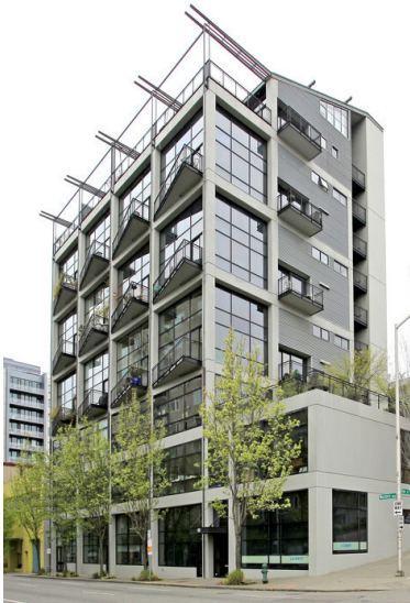
Wainstein A + U Architects, Banner Building Seattle, WA, 1993
