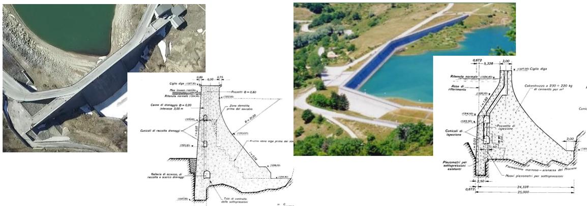
Figure 2. Rio Fucino gravity dam (on the left) and Sella Pedicate gravity dam (on the right)
