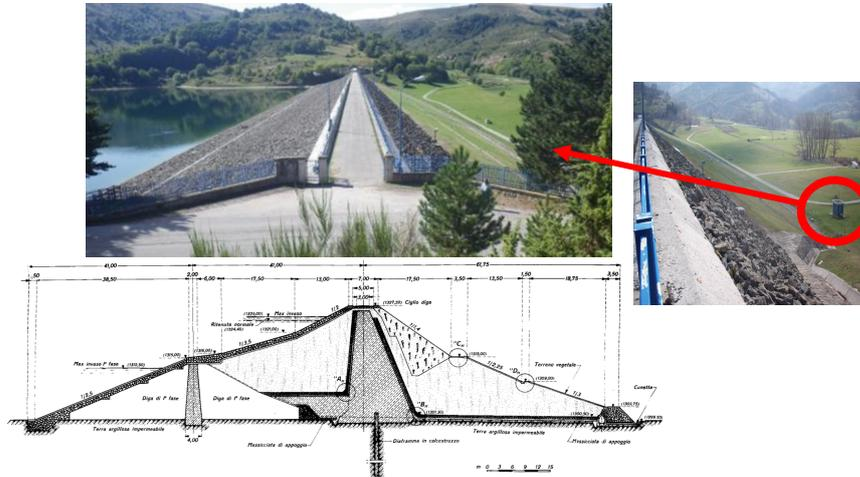
Figure 3. Poggio Cancelli embankment dam. The accelerometric station is shown on the right.
