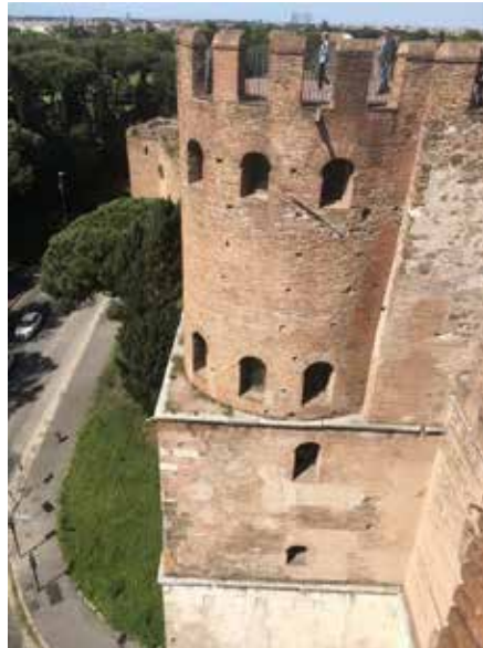
Fig. 3. Masonry of San Sebastiano Gate.
