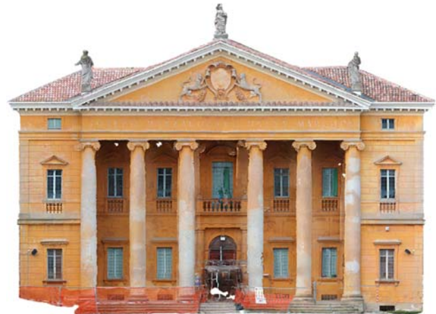
Figure 8. Ortho-mosaic of the building façade.
