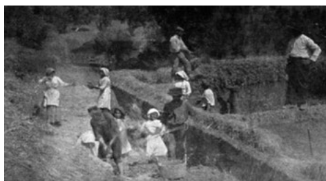
Fig. 2. The construction process involves the entire family, photograph of 1919 from a private archive
