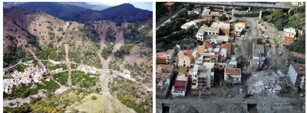
Figure 2. Damage to the infrastructures caused by the shallow landslides event that occurred in the Briga and Giampileri Villages on the 1 October 2009 and afterwards named the “Messina flood”.
