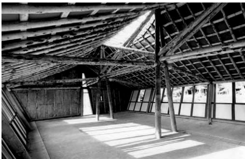
Fig. 10 | The 'Big Shed' Assembly Workshop (2012) by AA Design & Make with Mitchell Taylor Workshop and Atelier One (credit: V. Bennett, 2012).
