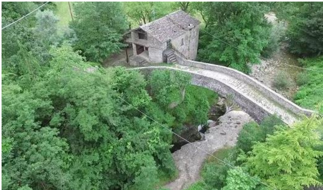
Figure 1: Aerial view of the bridge
