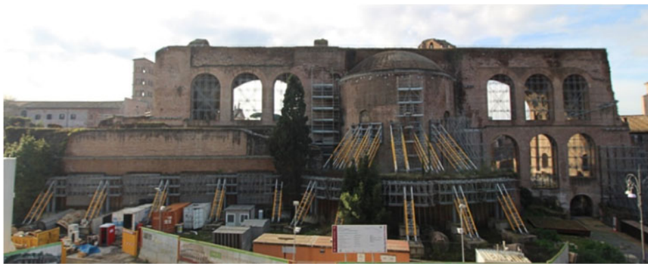
Figure 8. Temporary structural interventions installed on the Basilica.
