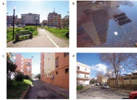
Fig. 1. Rione Marconi. (a) Open Space in the heart of the Area; (b) Damages to the sewing system; (c) Lack of maintenance; (d) School (Authors' photographs)
