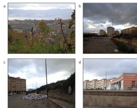
Fig. 2. Arghillà. a) View from the area; b) Lack of maintenance; c) Lack of services; d) Underutilized public spaces (Authors' photographs)
