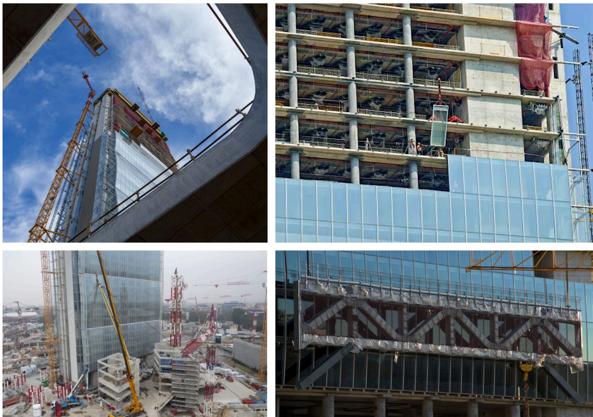
Figure 7.3: Worksite pictures of Isozaki tower under construction (2012-2015)
