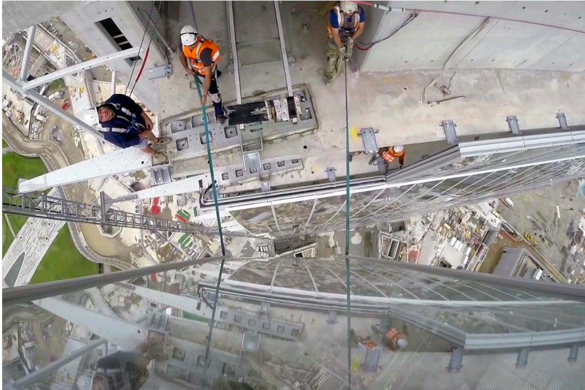
Figure 7.7: Worksite picture of on-site installation of the glazed modules. Source: https://www.focchi.it/it/
