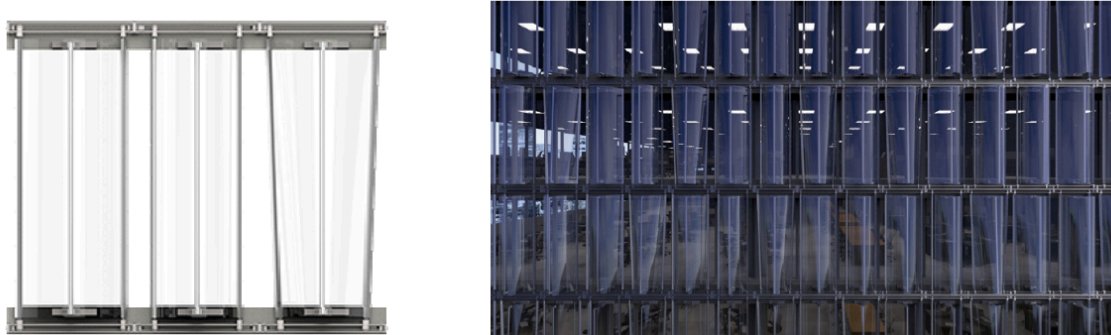
Figure 2.23: Adaptive thin glass facade model. Source: Ribeiro Silveira, R. (2016). Flexible transparency: a study on thin glass adaptive façade panels
