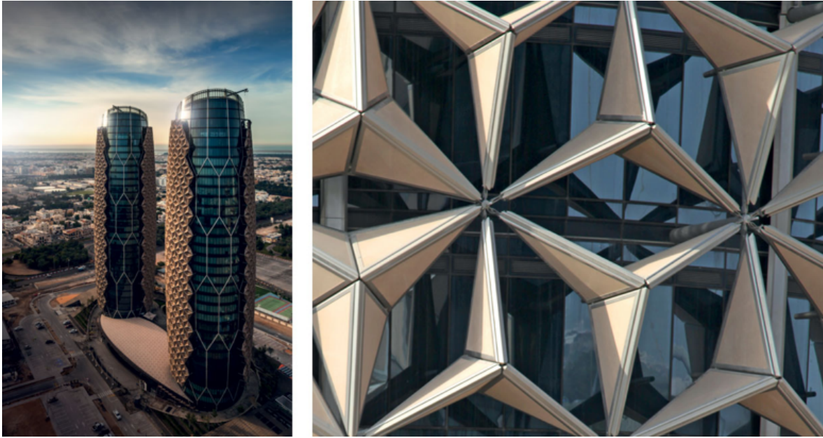
Figure 2.22: Intelligent adaptive envelope of Aedas Architecture’s Al Bahar Towers (Abu Dhabi, 2012) that opens and closes following sunrays
