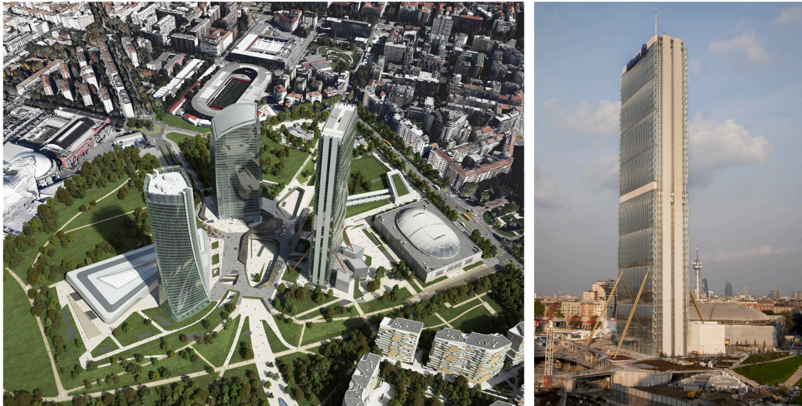
Figure 7.1: Isozaki tower located in the CityLife district of Milan, Italy
