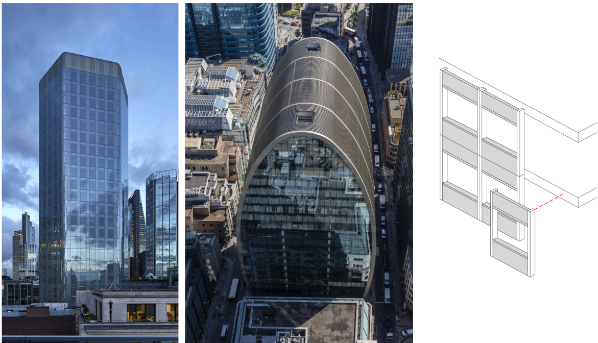
Figure 2.8: Assembly diagram and application examples of a unitized curtain wall system
