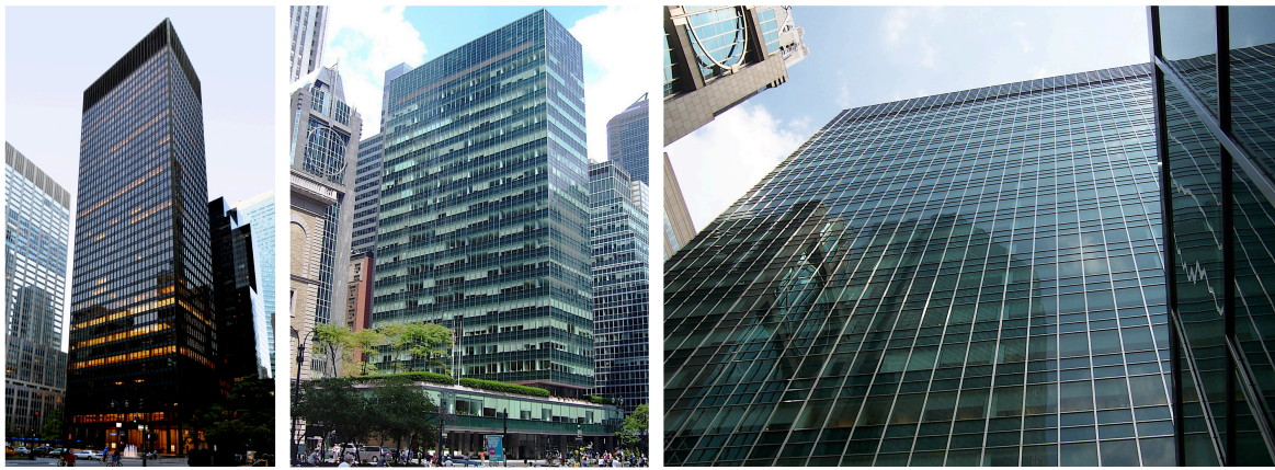
Figure 2.5: Curtain wall application on Lever House by Skidmore, Owings & Merrill (right) and on the Seagram Building by Ludwig Mies van der Roe (left)
