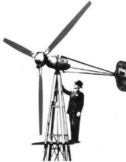
Figure 2.1. The Jacob's wind turbine [16]
