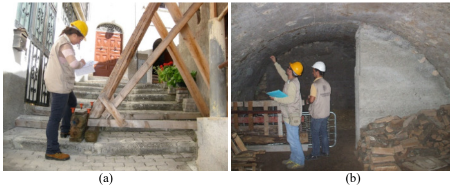
Figure 7: Students surveying structural features and damages of a building (a) and an hypogeal structure (b).
