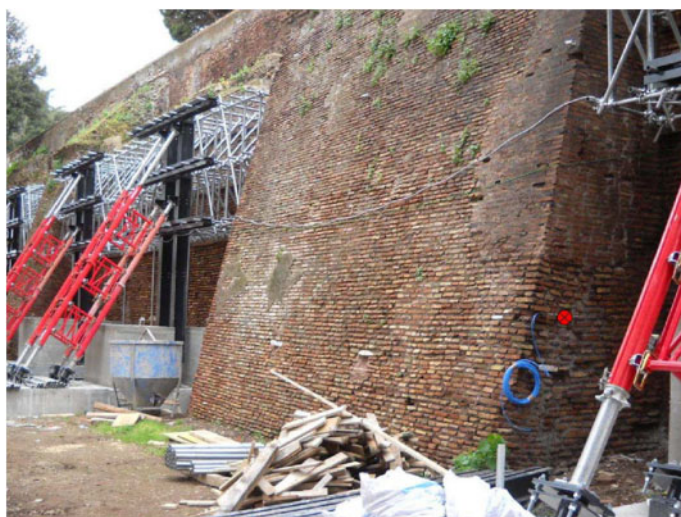
Figure 9. Temporary safeguarding interventions installed at the Aurelian Walls.
