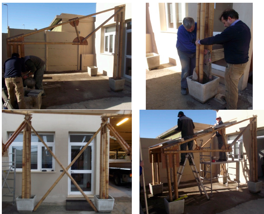
Figure 7. Assembly phases of the 1st full scale specimen.
