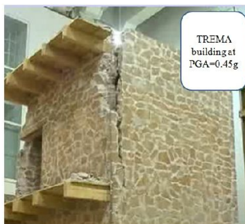
Fig. 8. The TREMA building at 0.45g: rocking of the upper wall
