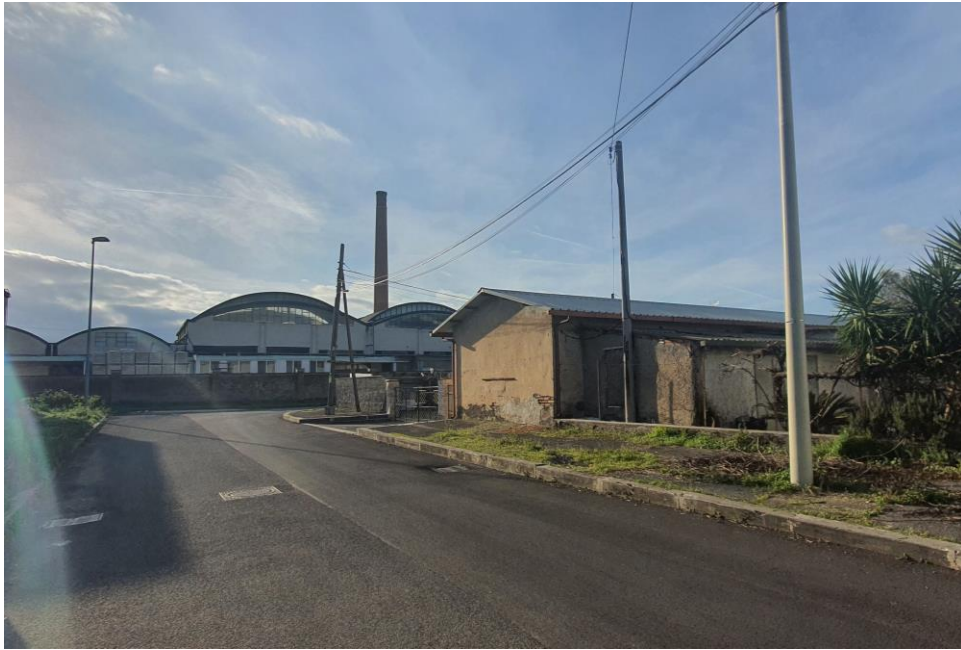
Figure (04-14) An example of the “ eternit ” roof in some structures in the industrial area in Pontinia. (taken by the Author). It is worth mentioning that the majority of the participants stated that “ eternity ” characterized the majority of the buildings (more than 90%) within the macro context of Pontinia. While the conclusion of the on-site investigation of the micro-context (limited to the inhabited center, 1 km 2 area) found another result, most buildings are constructed from conventional materials (reinforced concrete skeleton and brick).
