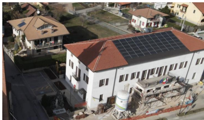
Figure (02-21) Installed PV on the municipality building in Magliano Alpi rural settlement (Magliano Alpi, 2021). The municipality led the implementation of a pilot project (top-down practice).
