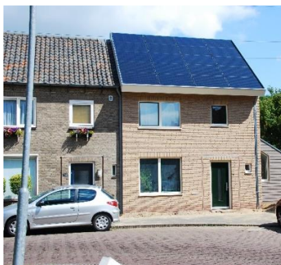
Figure (03-32) A retrofitted building in Den Bosch City, using an agile methodology (PassREg, 2015a).
