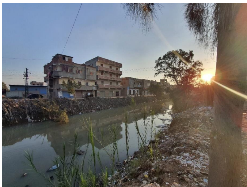
Figure (01-14) An exposed sewage canal for solid and agriculture wastes accumulates garbage on the canal banks. That has negative environmental and well-being impacts, and it promotes the spread of respiratory and epidemic diseases(taken by the author). The government is targeting the development of this canal.
