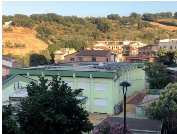
Figure (02-22) Some photovoltaic systems in the CER of Biccari, adapted from (Vidovich et al., 2021)
