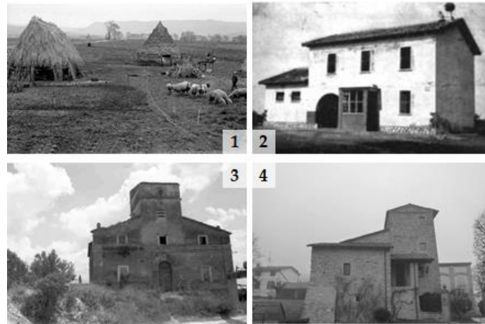
Figure (01-30) Traditional rural buildings typologies in the Lazio region. Panel 1: shows A single-room dwelling built with mixed clay and straw (Pontiniaweb, 2021). The huts present in southern Lazio are called “ Caprareccia .” Panel 2: shows Two-story houses with elongated shapes and several rooms built in stone (Borghidilatina, 2021). The house developed with the increase of family members and agriculture intensity. The houses also incorporate the services, such as stables and barn. Panel 3: shows a massive farmhouse (two-story construction) “ Casale .” (DIGILAND, 2021). There was a large courtyard where part of the livestock was housed. Panel 4: shows a four-story tower house, “ Casa a Torre ,” with massive fortification. (DIGILAND, 2021) Mixed-use building (residential, granaries, and stables ).
