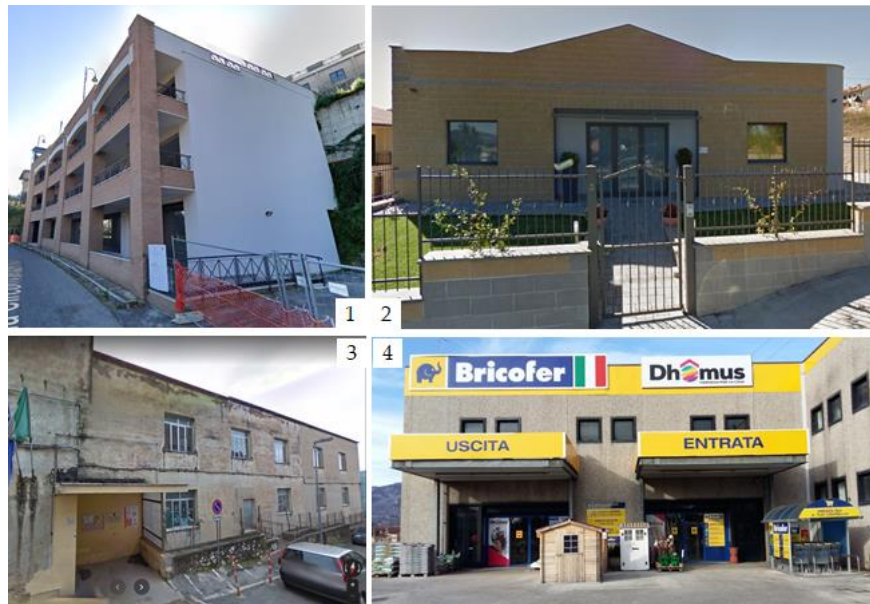
Figure (01-58) Some examples of service and commercial buildings in traditional settlements in the Lazio region (Google Maps, 2021). Panel 1 : shows a contemporary police station in Torrice, Frosinone. Panel 2 : shows a private medical center in Acquapendente, Viterbo. Panels 3 : depicts an elementary school in Roccagorga, Latina; the elementary schools in Lazio have the highest share by 40%. Panel 4 : shows a modern shopping store in Sant'Elia Fiumerapido. Services and commercial buildings are (11803 and 18979), demonstrating (8 and 13) % of the total non-residential buildings in Lazio.
