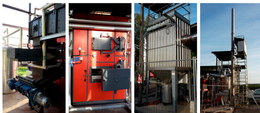
Figure 1. Details of the CHP plant (double screw mechanism, furnace, baghouse filter, and chimney).
