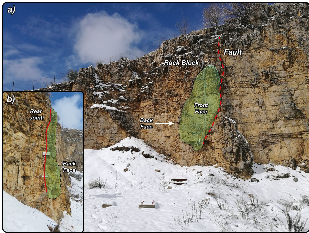
Figure 3.12. Front view of the potentially unstable rock block selected as the main target of the multiparametric monitoring system of the Acuto field laboratory, along with the fault line that laterally bounds its volume (a); Back view of the rock block and of the open joint that determines the its partial detachment from the rock wall behind.
