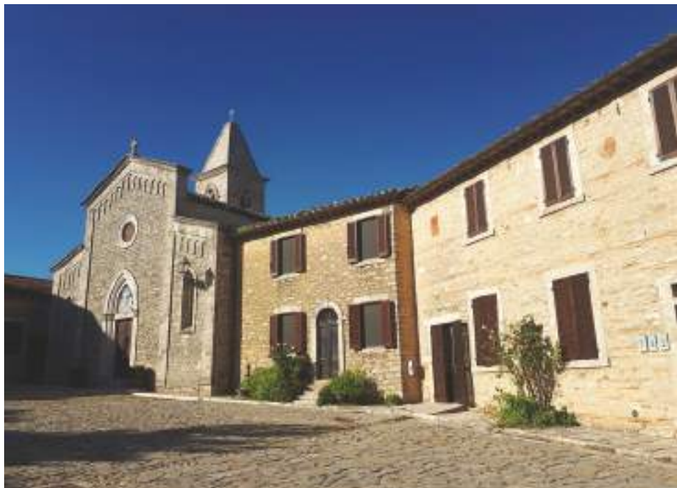
Fig. 28. The square in the centre of the castle. The restored medieval buildings. Photo by E. C., 2020.
