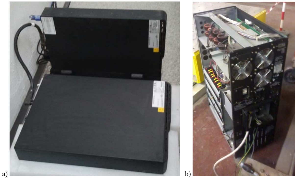
Figure 8. UPS - online double conversion type; a) P = 3 kVA; b) P = 10 kVA
