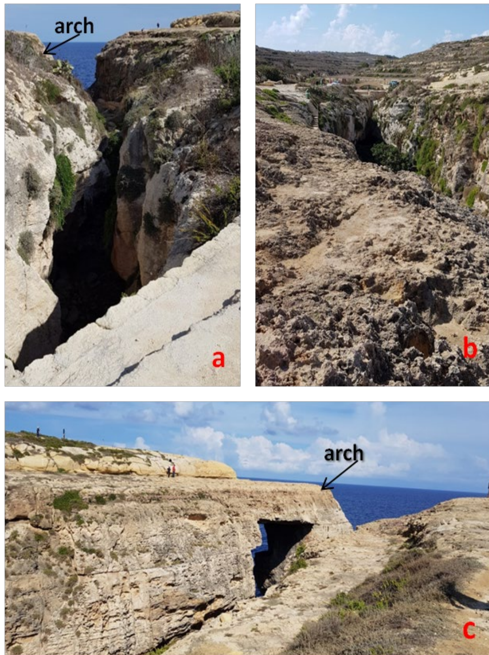
Figure 3. The figure shows the narrow, deeply engraved river valley, both in the terminal part (a) and upstream (b) of the natural arch of Wied il-Mielah with a rectangular vault (c).
