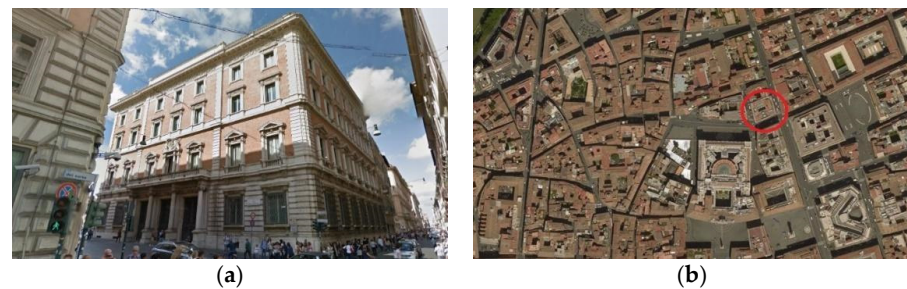
Figure 1. (a) Rome historic centre and case study building detail; (b) building view.
