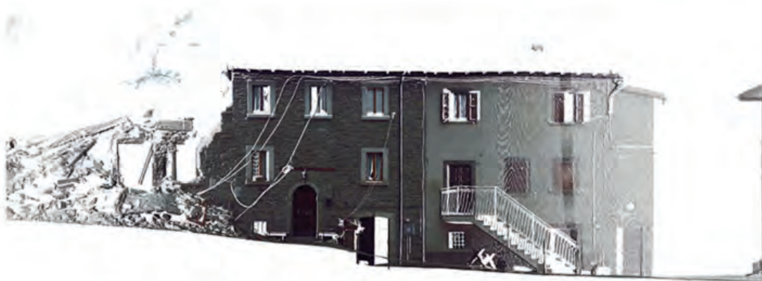
Grisciano Village, Ortophoto from laser scanner survey (L. Paris).
