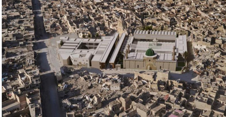
Figure 6. *Bird-eye view of the all complex.
