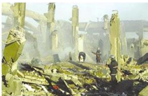
Figure 10. The accident in Skikda (Algeria) in 2004
