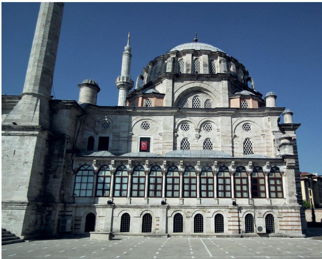
Fig. 5. Istanbul, Laleli Mosque (1759–1763), attributed to Mehmet Tahir Ağa. Detail of the Southwestern façade with arcatures, curvy transition profiles and portico. Photo A. Metin
