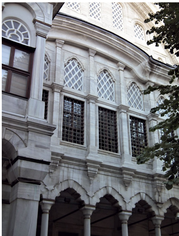
Fig. 1. Istanbul, Nuruosmaniye Mosque (1748–1755) by Simeon Kalfa. Detail of the Eastern façade with windows and portico arches with S and C profiles and elaborate curvy cornice. Photo A. Metin
