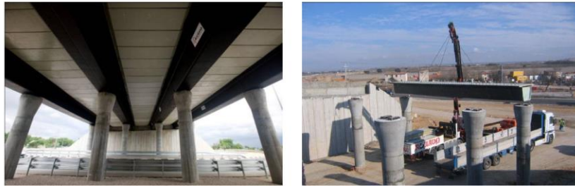
Fig. 1. Vehicular FRP bridges: M111 Madrid (Spain) freeway [13].
