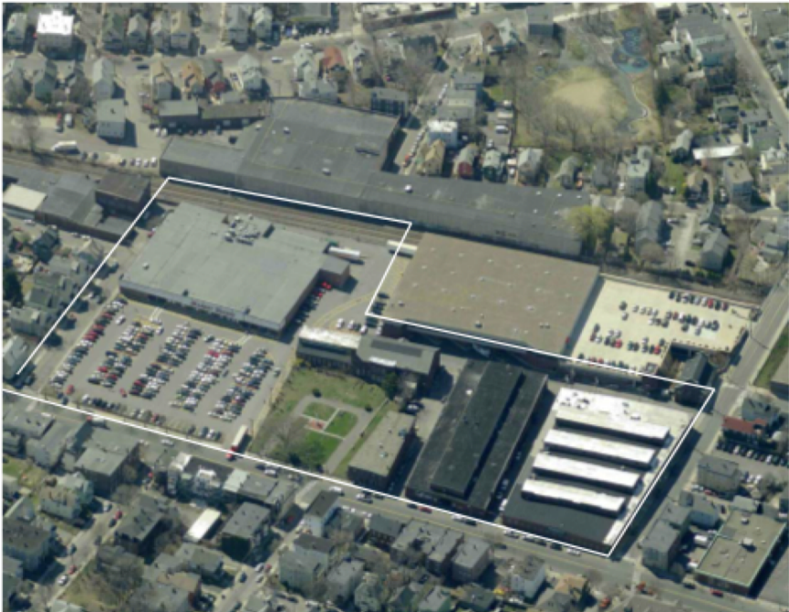
Figure 22 - Aerial picture of the location
