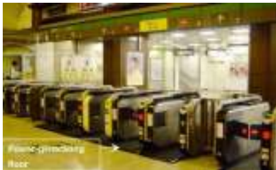
(b) Piezoelectric tiles installation at the Tokyo Station's Yaesu North Exit [Company 2008].
