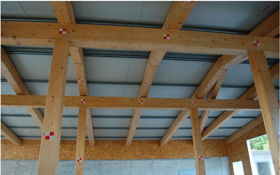
Figure 5. Monitoring system: detail of markers applied on the structure for the point detection
