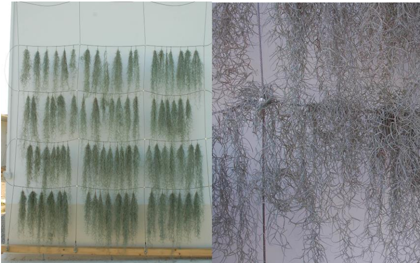
Figure 1. Left: assembled prototype of the steel mesh screen, with Tillandsia plants leaning against it. On the right, detail of the position of the plant on the prototype.
