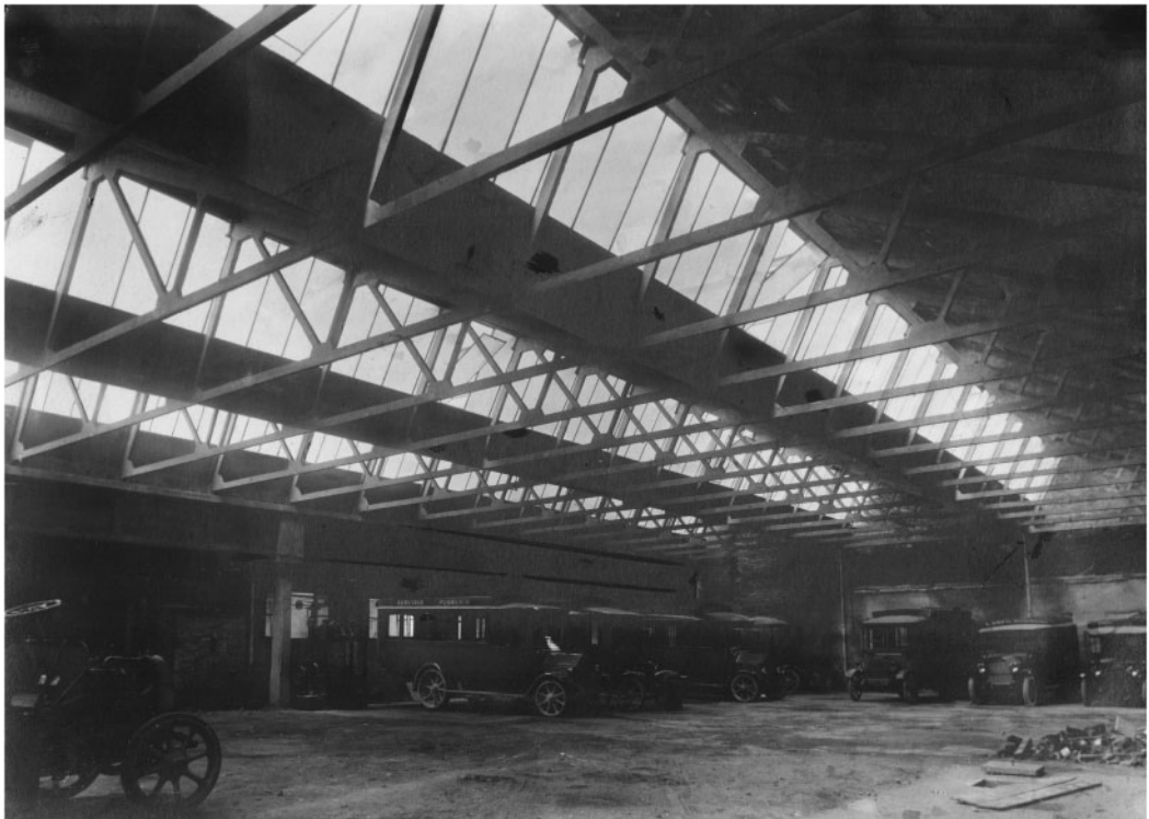
Figure 3. 1920, L. Santarella, Garage Fossati, Biella. Interior view of the roofing system (A. Bologna, private archive).
