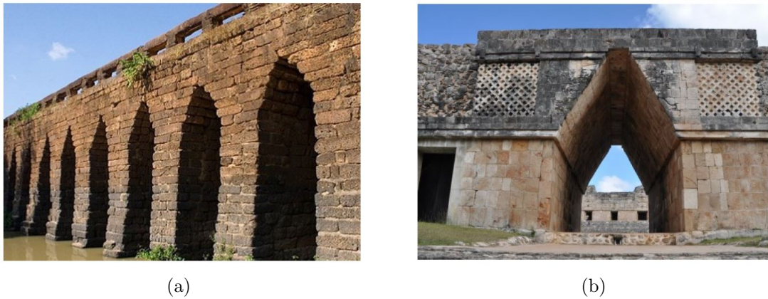
Figure 2.16: Some historical examples of a corbelled arch: (a) Kompong Kdei Bridge of Cambodia, (b) False arch at “Cuadrángulo de las monjas” at Uxmal in Yucatán - Maya architecture (from Iannuzzo (2018) ).
