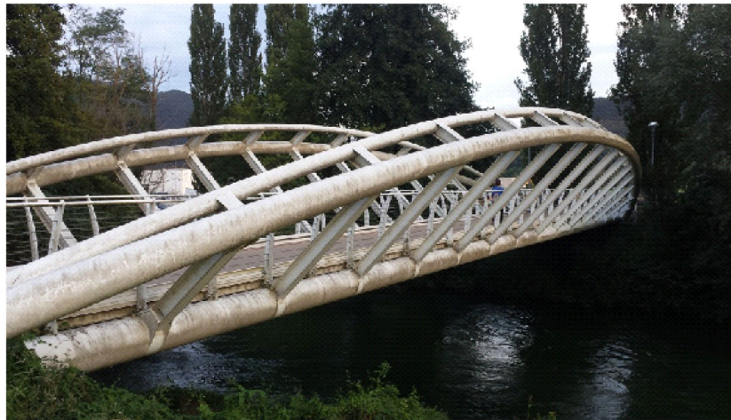
FIGURE 6 Picture view of the footbridge over the Velino River
