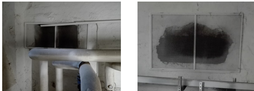
Figure 3.38: Tunnel entrances, at the foundations level, of the original heating system.
