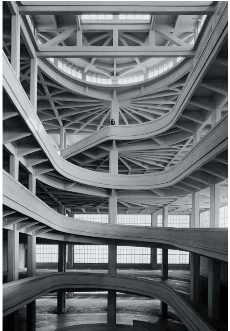
The northern helicoidal ramp of 1926 by engineer Giacomo Matté Trucco.
