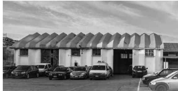
Fig. 11: Pier Luigi Nervi, Ferrocemento prototype in via della Magliana, Rome, 1945. View of the exterior (2017, photo by Fondi)
