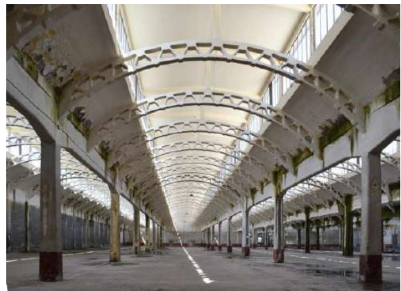
Fig. 5: Interior of the minor sheds (photo by Alexis)
