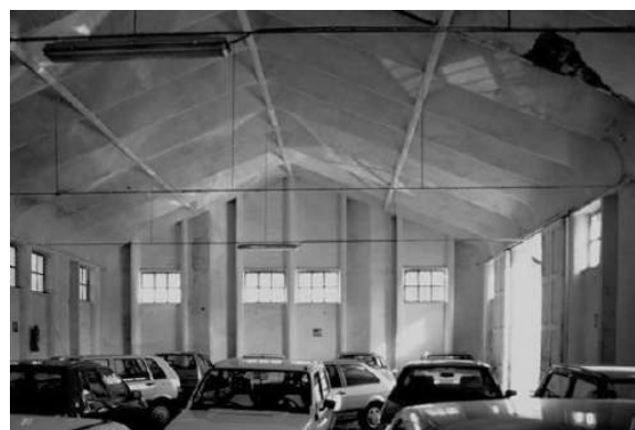
Fig. 12: Pier Luigi Nervi, Ferrocemento prototype in via della Magliana, Rome, 1945. View of the interior (2017, photo by Fondi)
