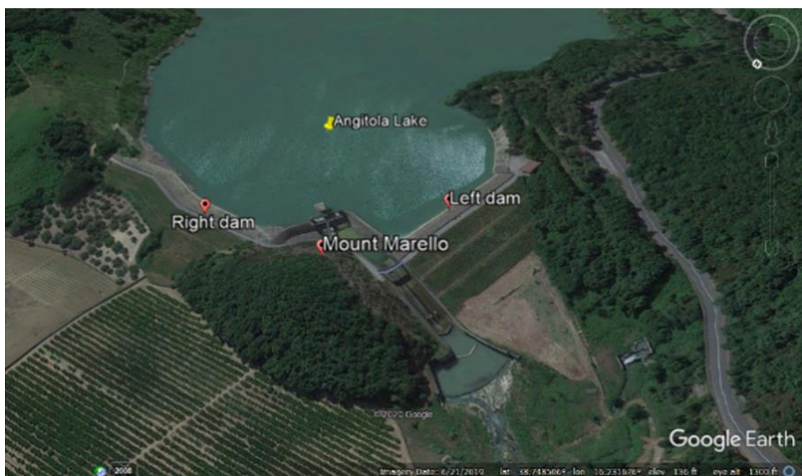
Figure 5.29: Aerial photo of Angitola reservoir in Calabria (Google Earth, 2019), Angitola lake; Monte Marello; Left and Right dams.
