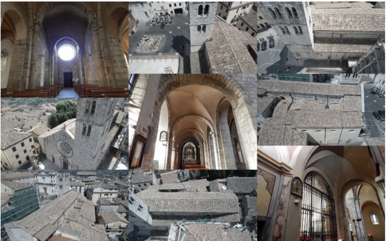
129 Figure 2 – Examples of photographs taken both using UAS and stationary cameras to produce a high-density point 130 cloud.
