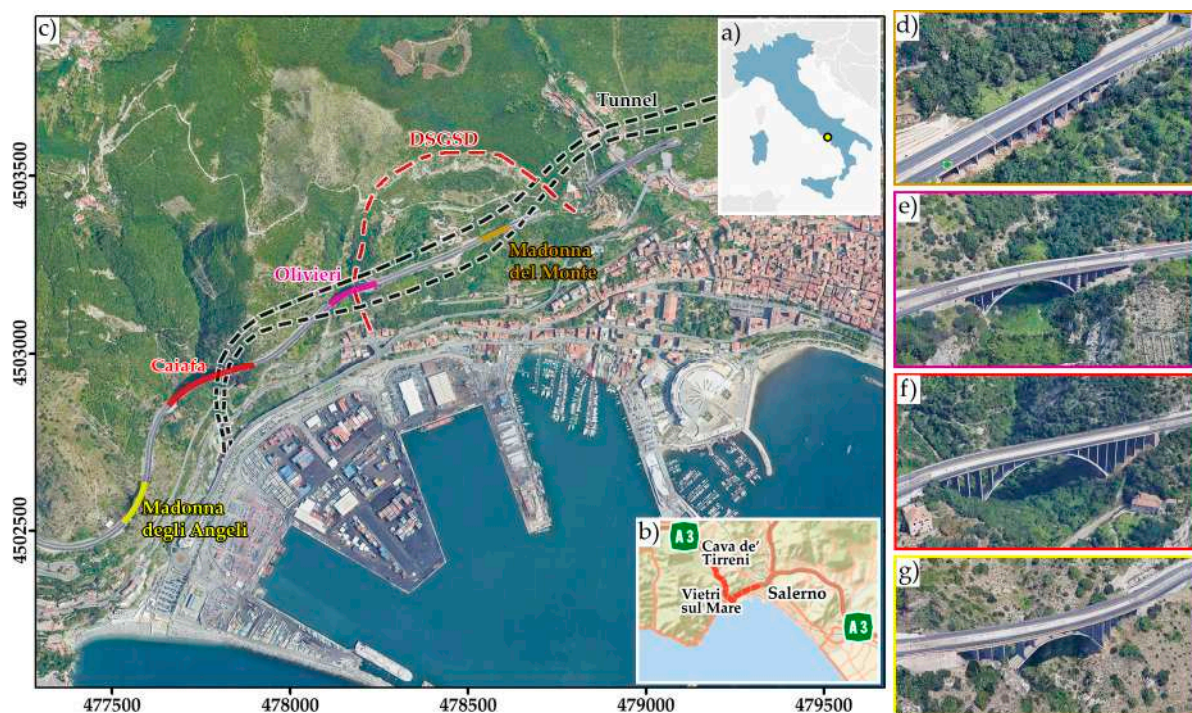
Figure 1. Focus area. (a) Map of Italy showing the location of focus area; (b) section of A3 highway analyzed; (c) excerpt of map showing the location of the four viaducts being analyzed, north of the Salerno port and (d–g) perspective views of the four viaducts in order: Madonna del Monte, Olivieri, Caiafa and Madonna degli Angeli.
