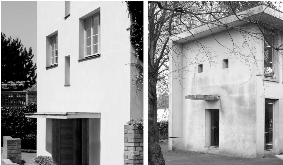
Fig. 1. Comparison between the facades of Adolf Loos’ Villa Muller in Prague and Álvaro Siza’s Carlos Ramos Pavillion in Oporto
