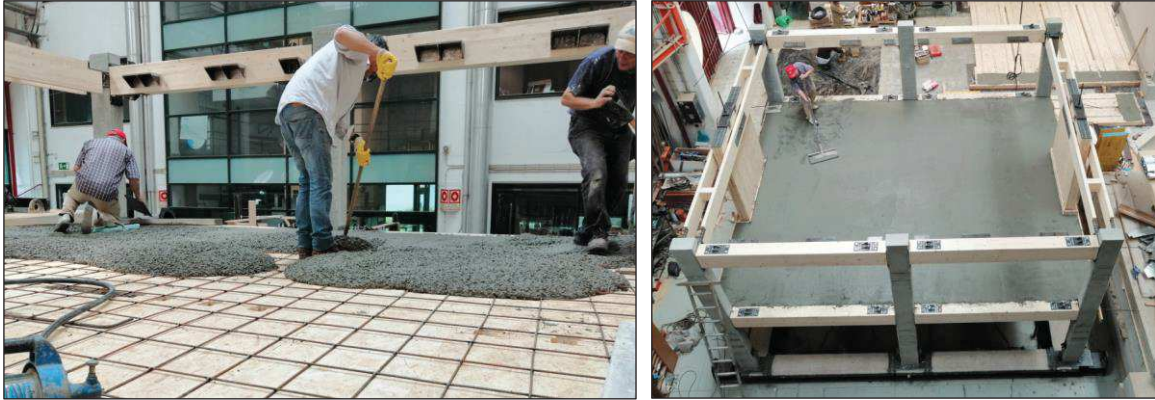
Figure 6.25. Phase 4b: Casting of the concrete slab.
