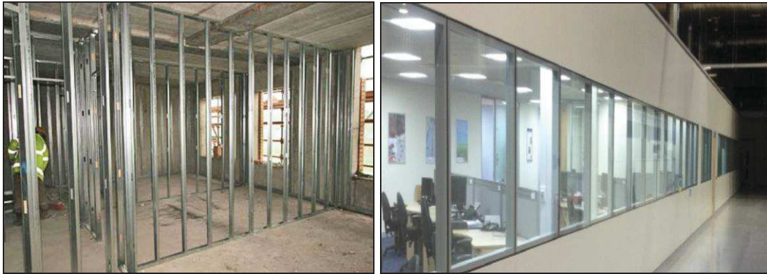
Figure 2.26. Examples of metal partition walls (source: www.diy-extra.co.uk ).
