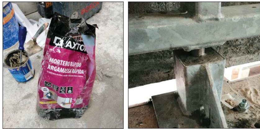
Figure D.15. Filling of the bottom anchorages using fast-setting mortar.
