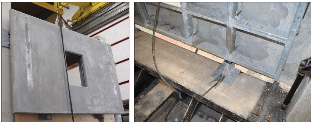
Figure D.11. Checking the position of the panels in the upper level (left) and fixing of the anchorage devices to the specimen foundation (right).
