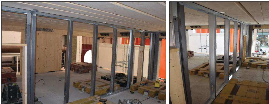
Figure 6.29. Construction of the steel sub-frame.
