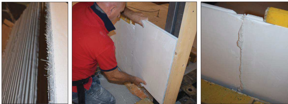
Figure 6.32. Detail of the fiber-reinforced gypsum panel (left) and assemblage of the panels through male-female joints (centre) and additional glue (right).
