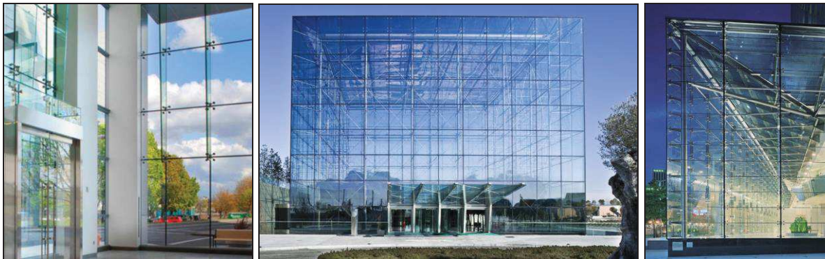
Figure 2.7. Examples of spider glazing systems (source: www.glasxperts.com , www.neelkamalfacades.com ).
