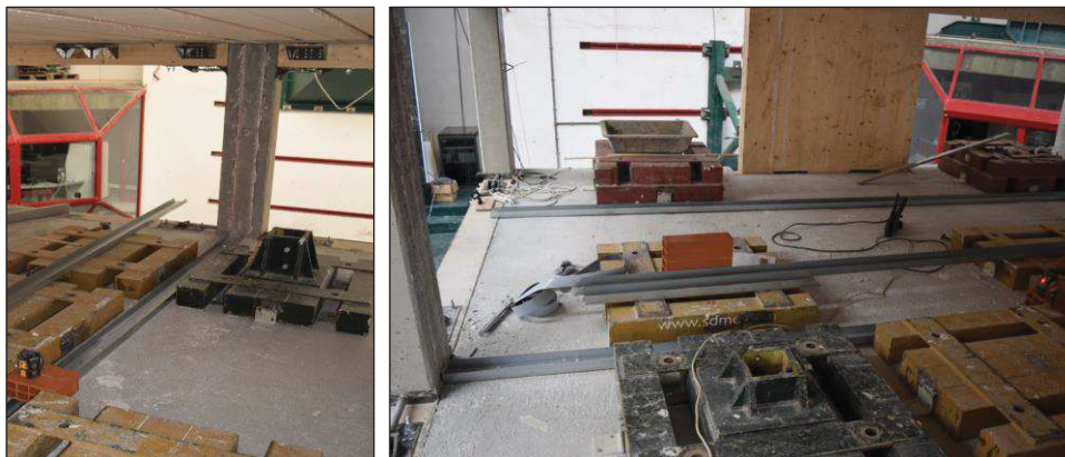
Figure D.22. Measurement of the horizontal alignment on the South (left) and on the North (right) sides before constructing the internal wall.
