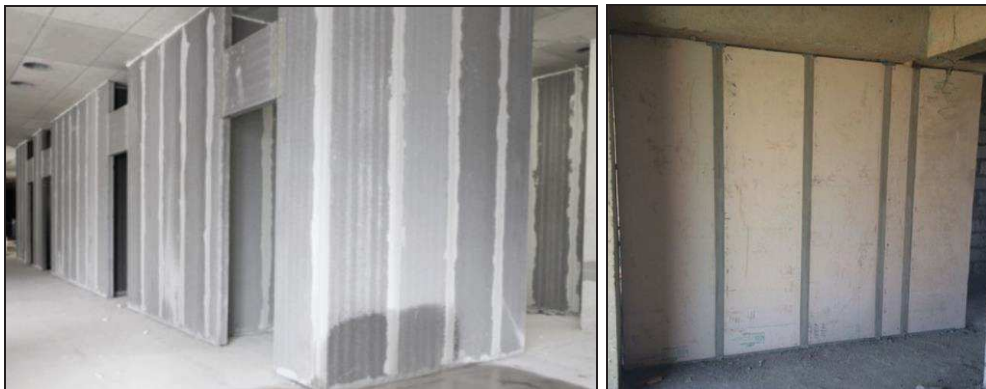
Figure 2.25. Examples of concrete partition walls (source: www.gharpedia.com ).
