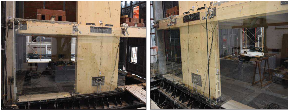
Figure D.20. Assembly of all the first level of the East-side façade: connection of the South-side panel (left) and of the North-side panel (right).
