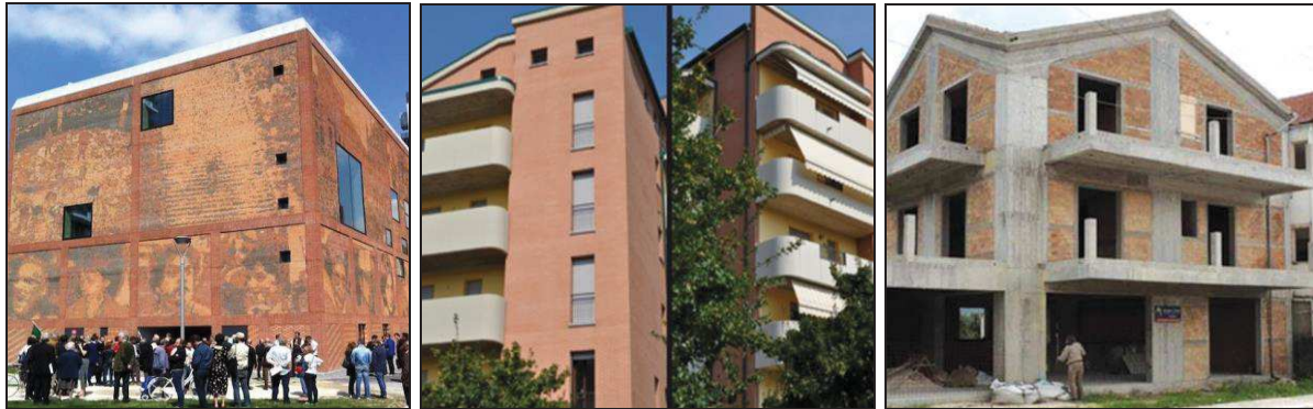
Figure 2.17. Examples of masonry infill walls (source: www.structuremag.org ).
