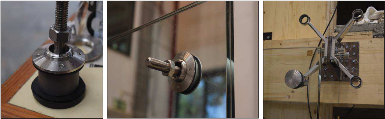
Figure 6.40. Connection of the rotules to the glass panels: particular of the rotule covered by adhesive tape (left), insertion of the rotule into the hole of the glass panel (centre), rotule/spider/plate connection (right).
