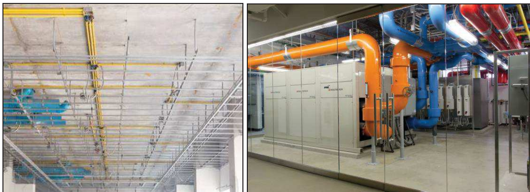
Figure 2.33. Examples of building services and contents (source: www.benincaprogetti.it ).
