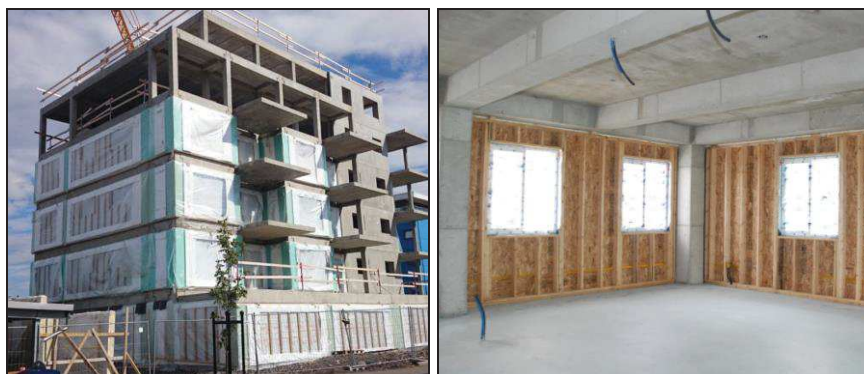
Figure 2.18. Examples of timber infill walls (source: www.canadawood.org ).
