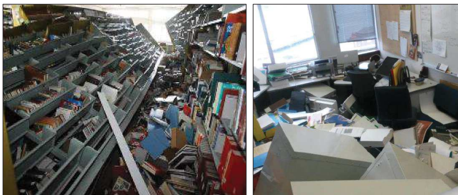
Figure 3.12. Damage to building contents (left: Dhakal 2010; right: Baird and Ferner 2017).
