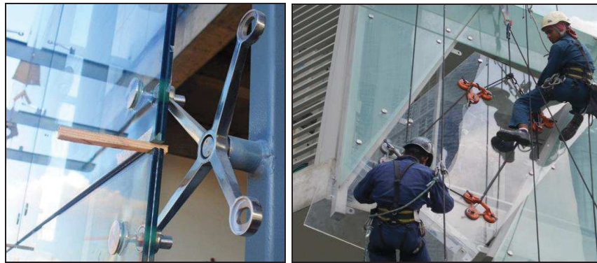
Figure 2.8. Spider glazing system: example of connection to the primary building and installation of the façade (source: www.glassarchservicesng.com ).
