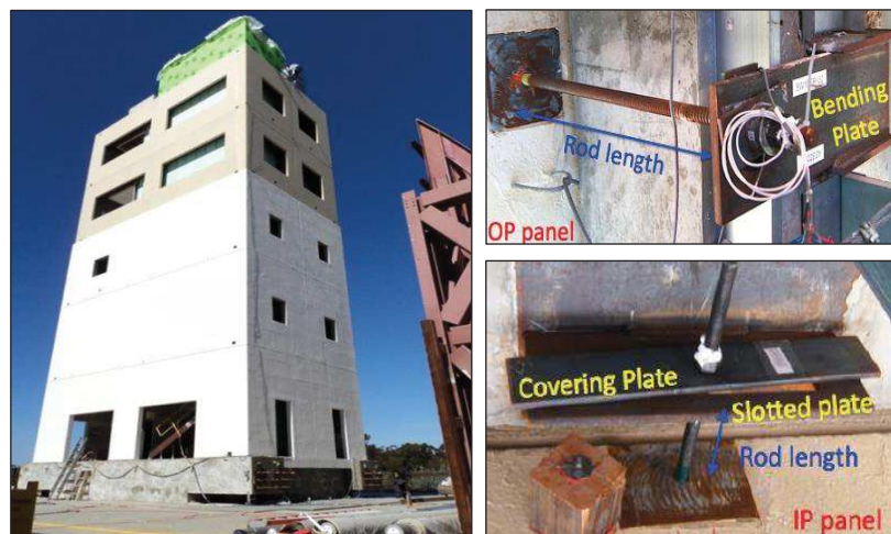
Figure 3.15. Five-storey Test Building (left) and cladding system details (Pantoli et al. 2013).
