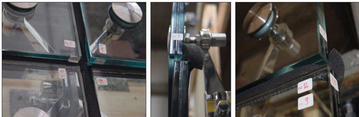
Figure 7.39. Measurements of the out-of-plane movement of the panels after all the testing sequence.
