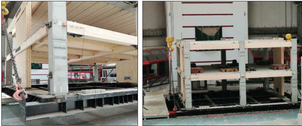
Figure 6.27. Lifting of the Test Building (left) and positioning on the shaking table (right).
