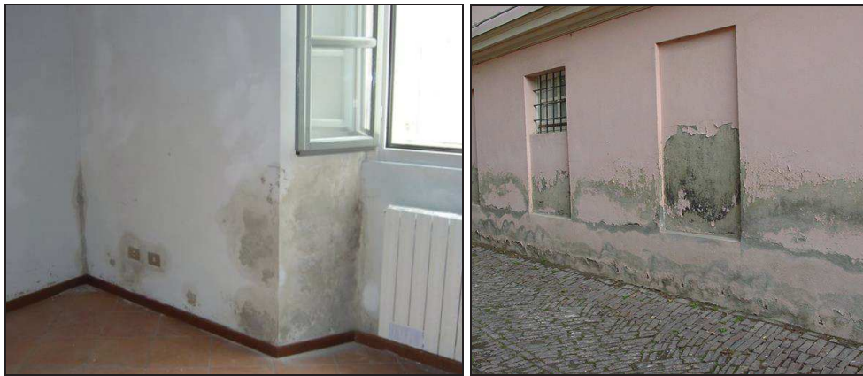
Figure 2.37. Damage to non-structural components due to temperature load (source: www.emmetisistemi.it ).
