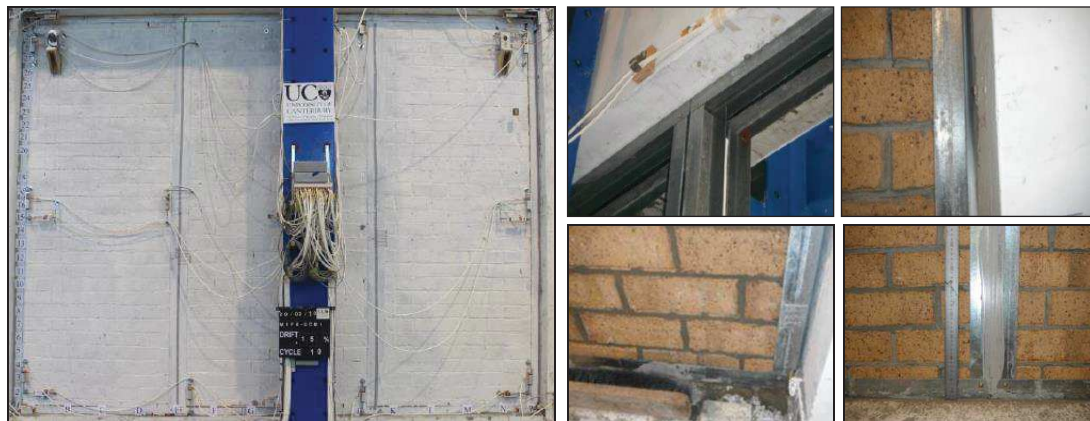
Figure 4.8. Left: Low-damage rocking infill wall (Taslignedik 2014); Right: construction details (top-left: sub-frame system; bottom left: clay bricks infilled within the sub-frame; top-right: polyurethane foam in the lateral gaps; bottom-right: polyurethane structural joint sealant into the lateral gaps) as described in Taslignedik (2014).
