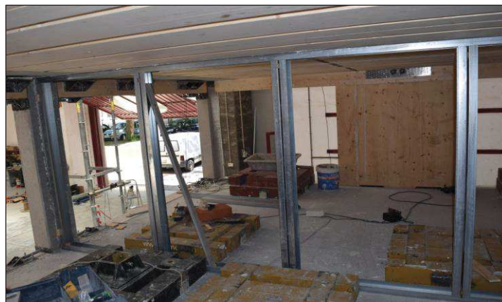
Figure D.24. Final configuration of the steel sub-frame.
